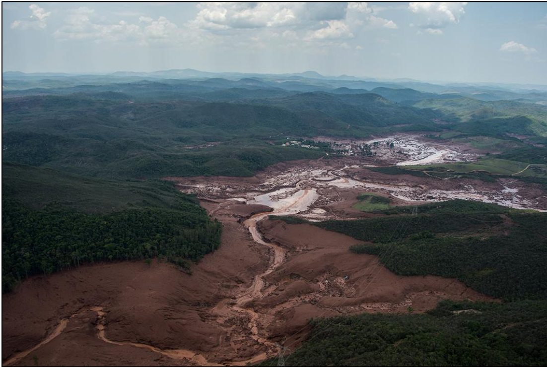
Figure 41. Example of the landscape effects of a TSF failure in Brazil
