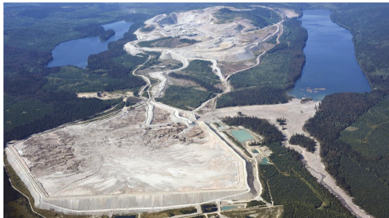
The empty tailings pond of Imperial Metal's Mount Polley mine following a dam breach. Toxic process water and mining waste flowed into nearby Polley Lake and down Hazeltine Creek.
